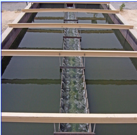
Tertiary Treatment Multi Media Filters above and Settlement Tank right
